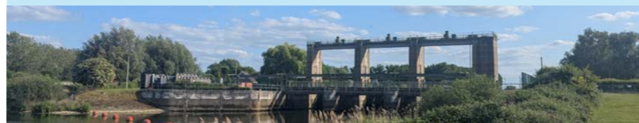
Figure 5. Sluice Gates at Denver
